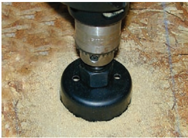
2. Drill hole in floor using hole saw.
